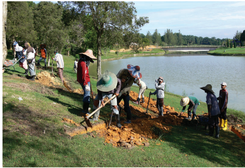
Digging drains, Malaysia
