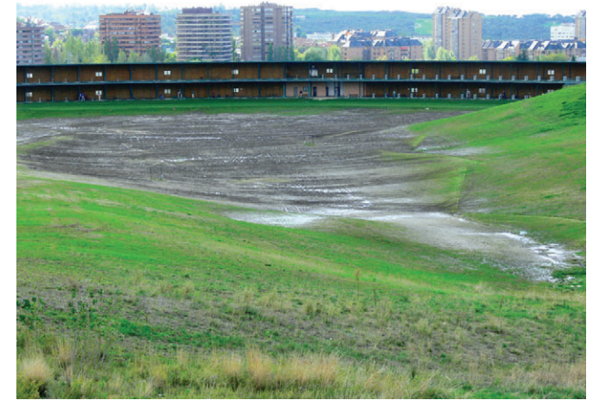
Poor drainage reduces potential revenue
